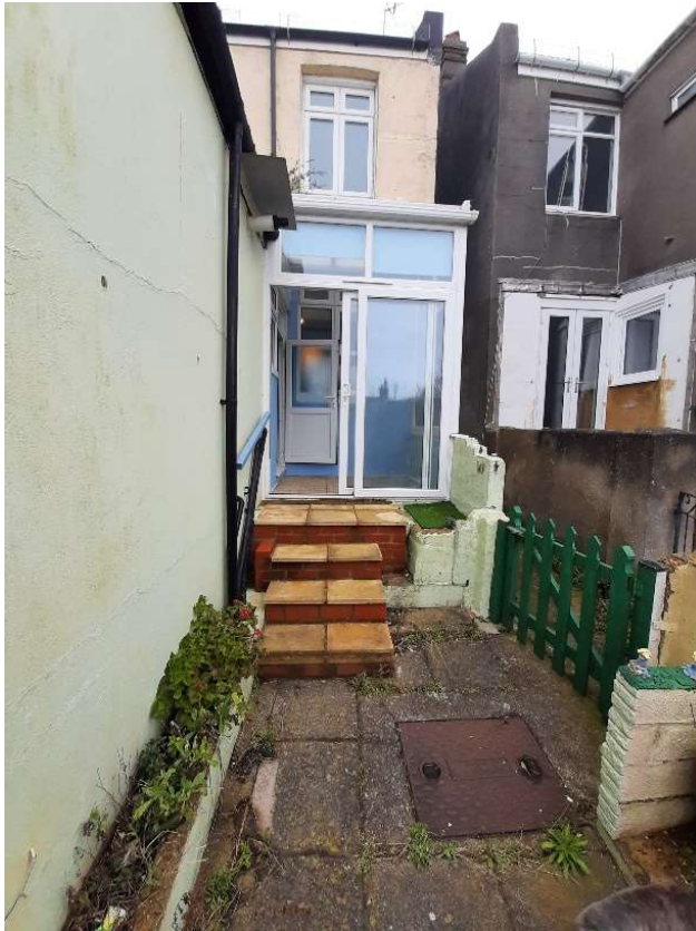
Existing conservatory in context with rear projection at no. 50.
